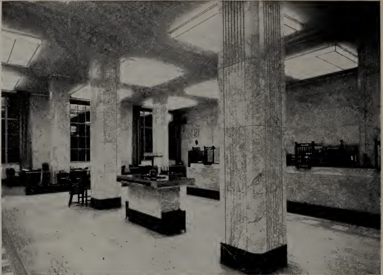
A SECTION OF HEAD OFFICE BANKING ROOMS 111 Franklin Street
